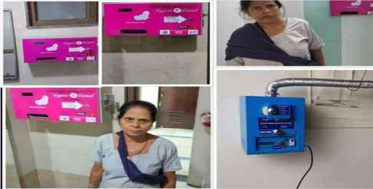
Installation of Sanitary Napkin Vending and Incinerator Machines
